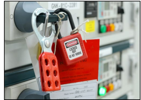
Figure 2 Safety Lockout in place. Tag and Lock styles may vary.
